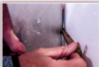
10mm graduated wedge used to check offsets (must be < 10 mm)
